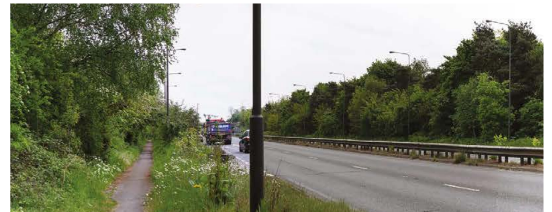
Figure 88. A23 Footway Looking South-East
